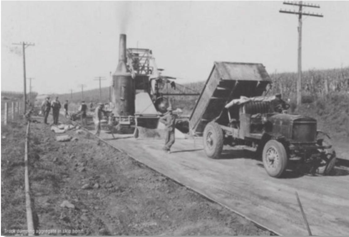
Truck dumping aggregate in skip hoist.
