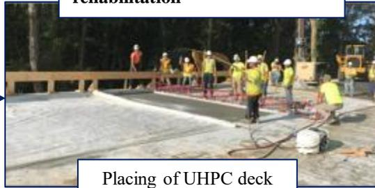
Placing of UHPC deck overlay
