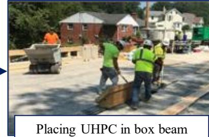
Placing UHPC in box beam connections
