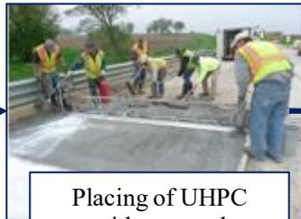
Placing of UHPC with a screed
