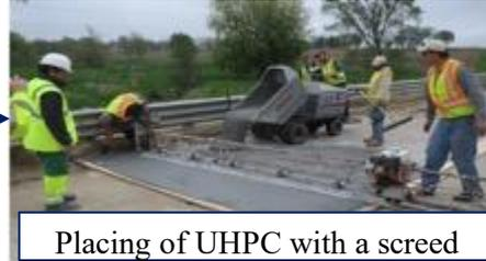
Placing of UHPC with a screed
