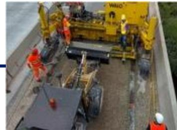
Unloading of the UHPC to the resurfacer
